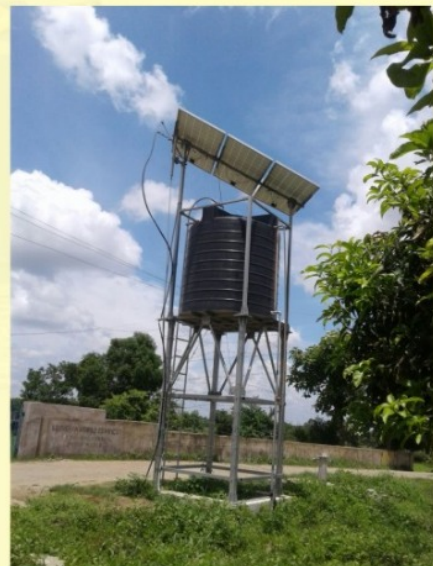
Actual Solar Water pump System Setup in Balangir Dist. of Odisha State
